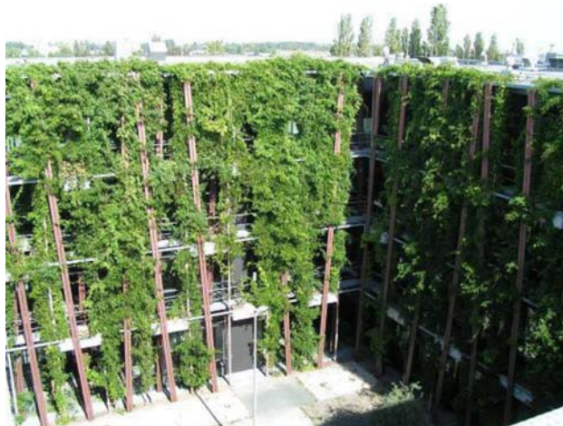
Figure 8 Façade greening system (priority 2)
