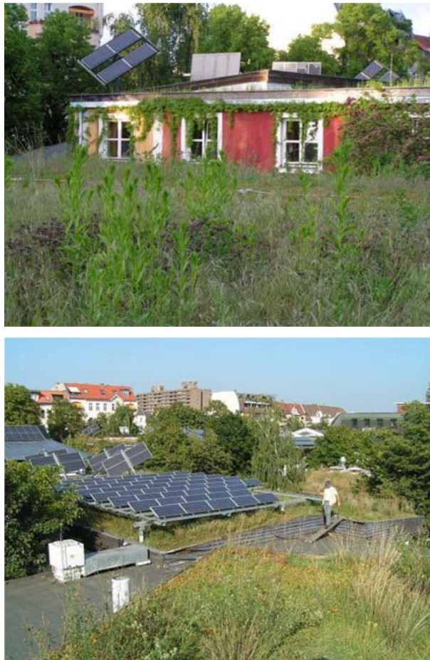
Figure 5 Greened roofs, UFA-Fabrik Berlin-Tempelhof (priority 2)
