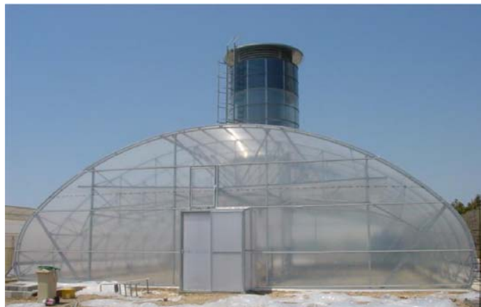
Figure 14 The Watergy prototype in Almeria (Spain), cooling tower in its centre (right)
