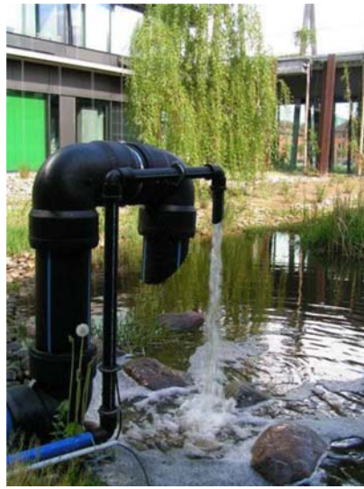
Figure 9 Artificial rainwater pond (priority 3) combined with trough infiltration for stormwater management (priority 7)
