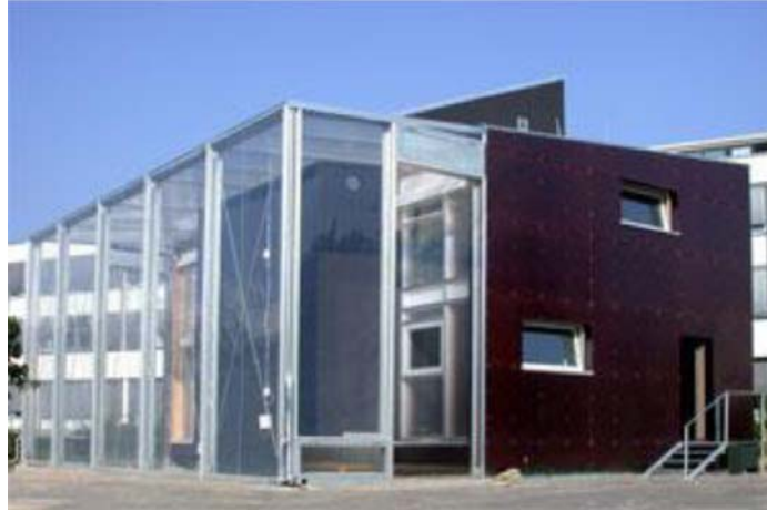
Figure 13 The Watergy prototype in Berlin-Dahlem (Germany), south-facing greenhouse façade
